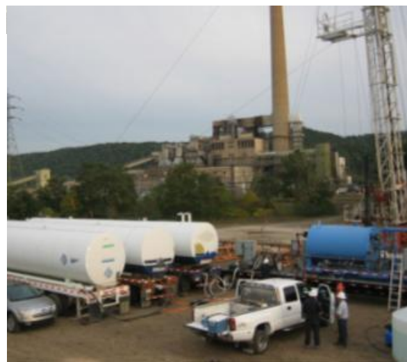
Injection Testing, October 2008
